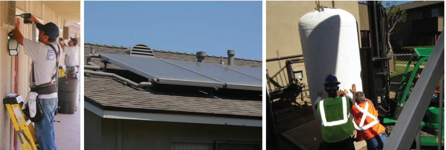
Left: New exterior CFL lighting was installed outside each apartment in May 2012. Center: Solar panels collect energy to heat the newly installed solar domestic hot water (DHW) system. Right: Installation of a new, insulated, 500-gallon water storage tank, which will hold the pre-heated water generated by the solar DHW system. Photography courtesy of LINC Housing; photos left and center by Gary Krueger Photographer
