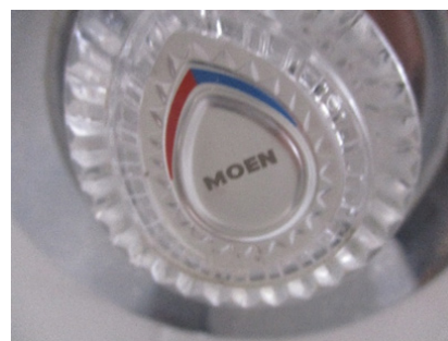
Figure 3. Moen Push/Pull shower valve containing a Moen 1200 cartridge. Unless the cartridge has been replaced with a Moen 1225 cartridge, it can be assumed all Moen shower valves contain Moen 1200 cartridges.
