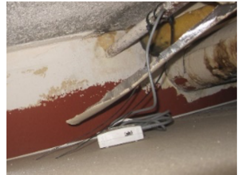
Figure 4. Temperature Data Logger Monitoring a Return Riser
