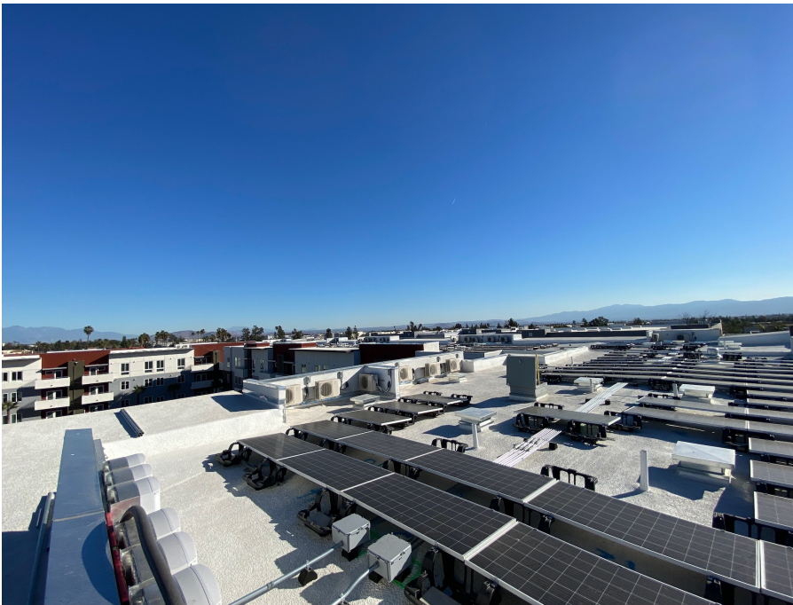
Well managed Roof for PV
